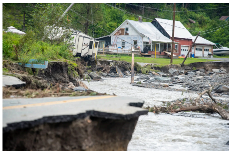
Extensive damage to Red Village Road in Lyndon is seen on July 31, 2024. File photo by Jeb Wallace-Brodeur/VTDigger
